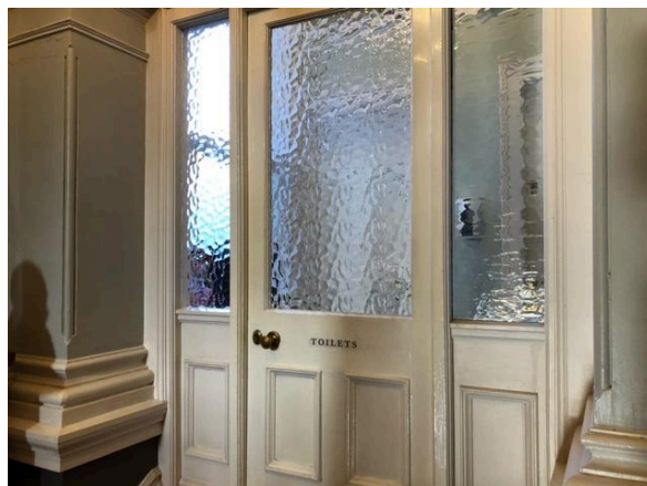
Image: First Floor Landing Toilets
